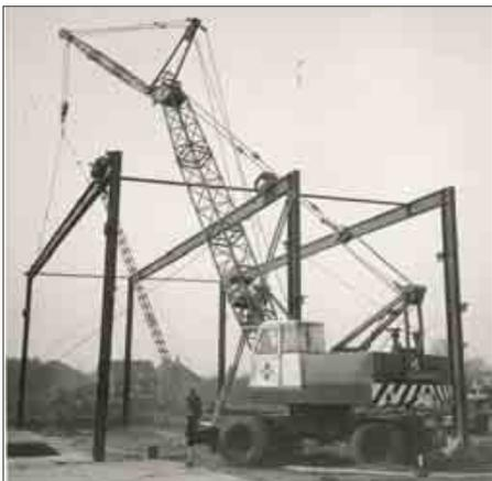
1972: Rope-driven SK 15 with plastic operator cab
